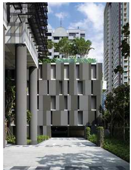
N°8 The entry to the car park, located below the environmental deck.
